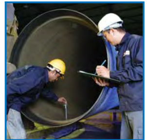
10. Internal Concrete Lining
