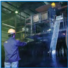
9. External Bitumen Coating
